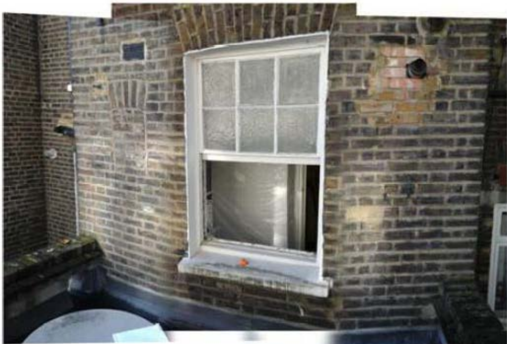
Terrace/ rear wall
