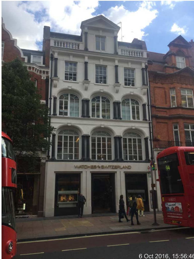
Oxford Street Frontage (Top) and North Row entrance to upper floors (Bottom)
